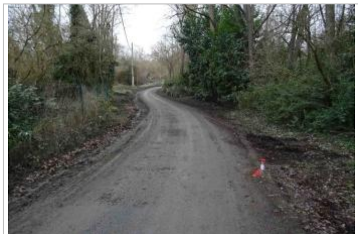
Photo repère © GEOSPHAIR
