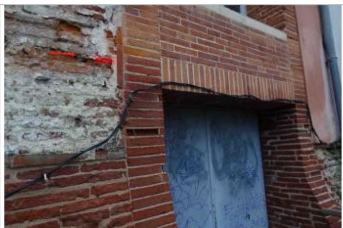
Photo repère © GEOSPHAIR
