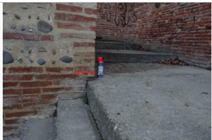
Photo repère © GEOSPHAIR
