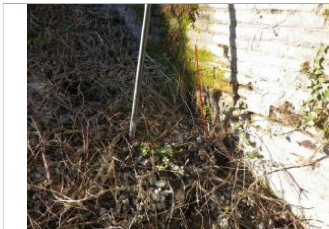
Photo repère © GEOSPHAIR
