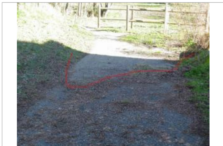
Photo repère © GEOSPHAIR
