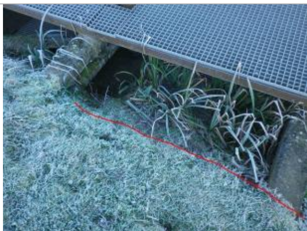
Photo repère © GEOSPHAIR
