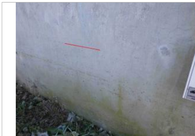
Photo repère © GEOSPHAIR
