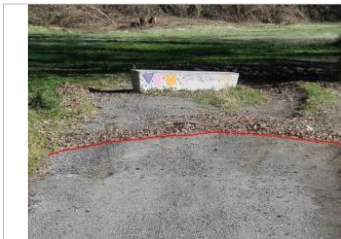
Photo repère © GEOSPHAIR
