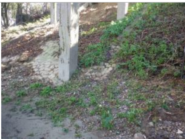
Photo repère © GEOSPHAIR
