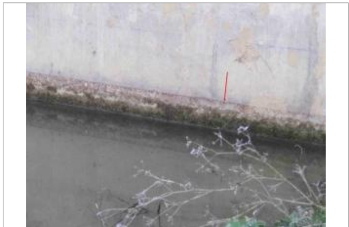
Photo repère © GEOSPHAIR
