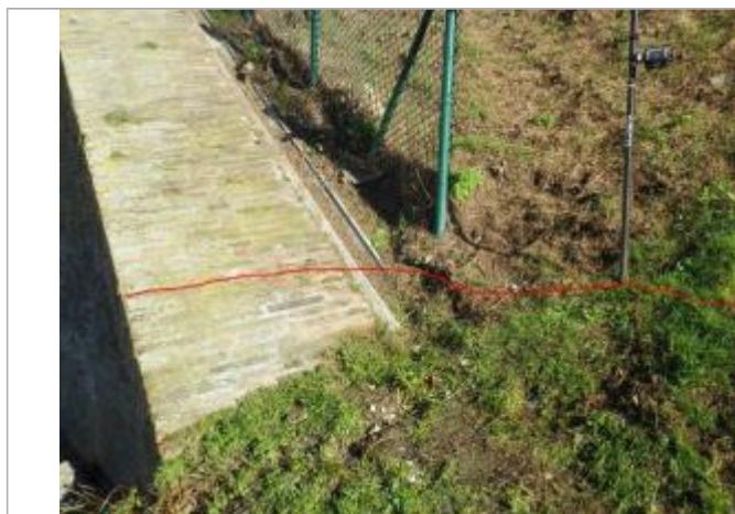
Photo repère © GEOSPHAIR
