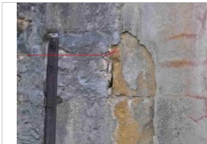
Photo repère © GEOSPHAIR
