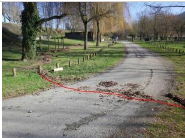
Photo repère © GEOSPHAIR
