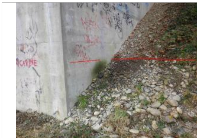
Photo repère © GEOSPHAIR
