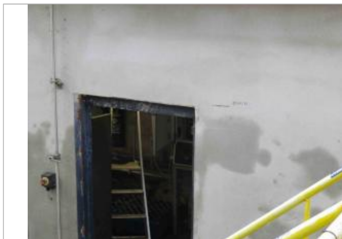
Photo repère © GEOSPHAIR
