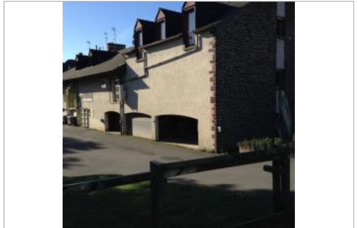
Parking atelier réparation proximi - garage
