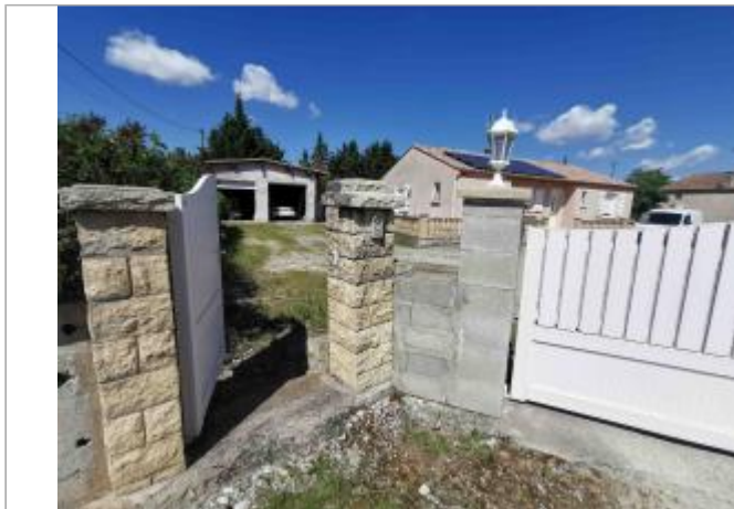
Garage - Photo © AGERIN
