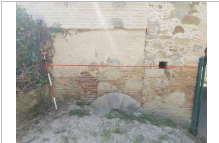
Batiment moulin - Photo © AGERIN
