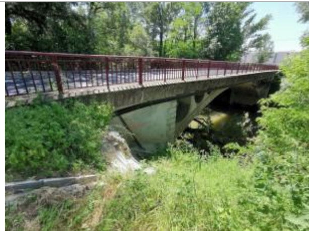
Pont (aval rive droite) - Photo © AGERIN
