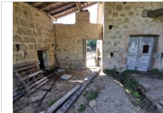
Batiment moulin - Photo © AGERIN
