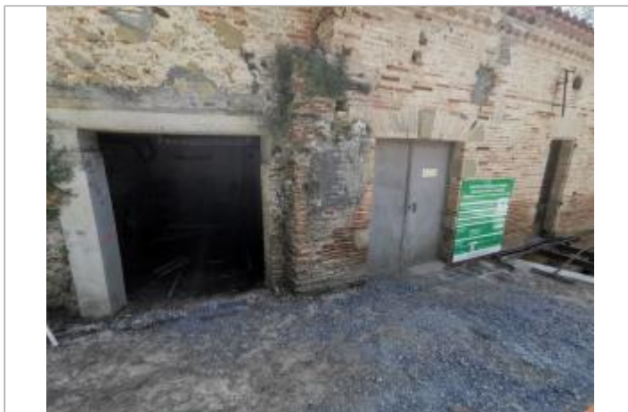
Batiment moulin - Photo © AGERIN
