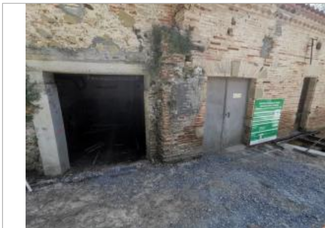
Batiment moulin - Photo © AGERIN
