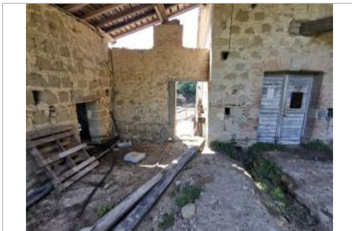
Batiment moulin - Photo © AGERIN
