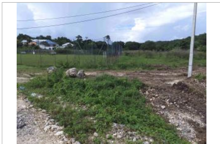
Inondation terrain de football
