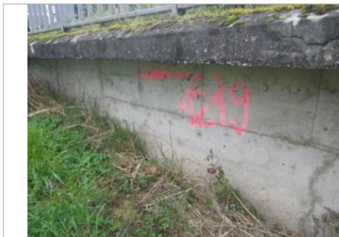
Trace mur quai - Photo ©AGERIN
