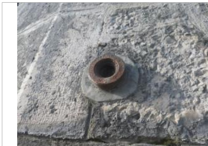
Plaque muret pont - Photo ©AGERIN
