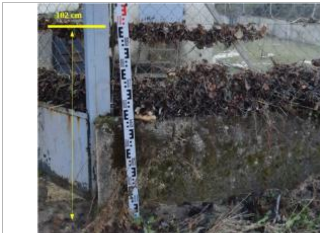
Grillage de la station AEP - Photo ©SBGH
