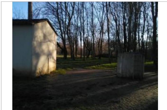
Station de pompage Condoumines - Photo ©AGERIN
