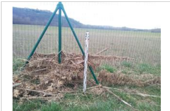
Station de captage - Photo ©AGERIN
