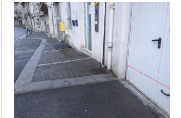
Photo repère © Survey
