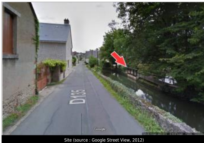
Site (source : Google Street View, 2012)
