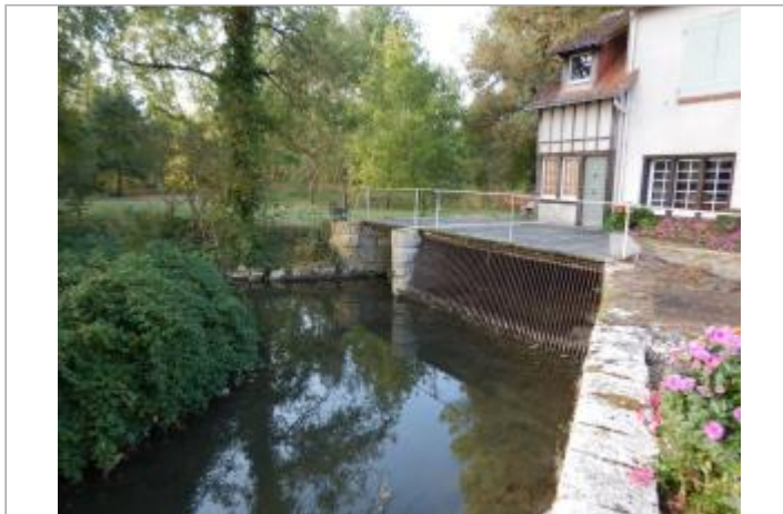
Site (source : SPC LCI)
