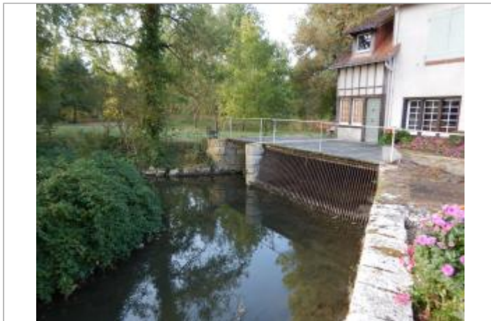
Site (source : SPC LCI)
