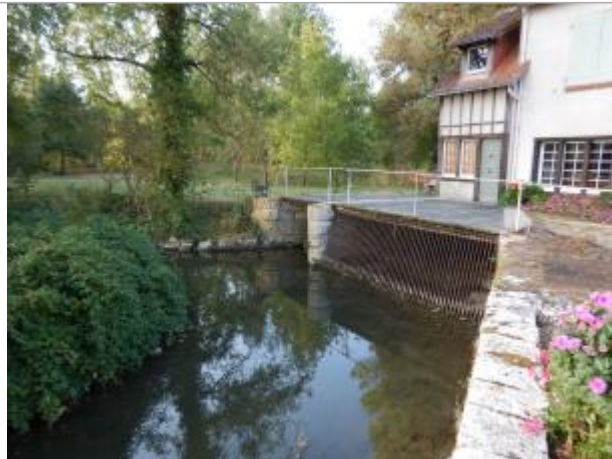
Site (source : SPC LCI)
