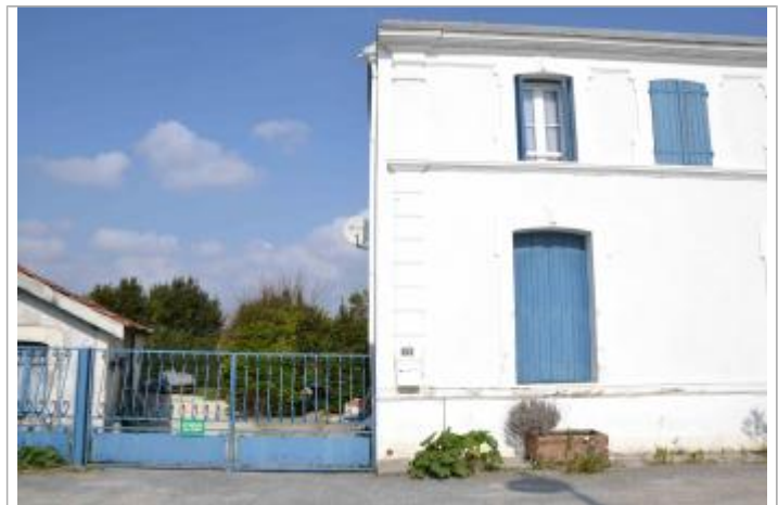
Repère Xynthia place Chatressac
