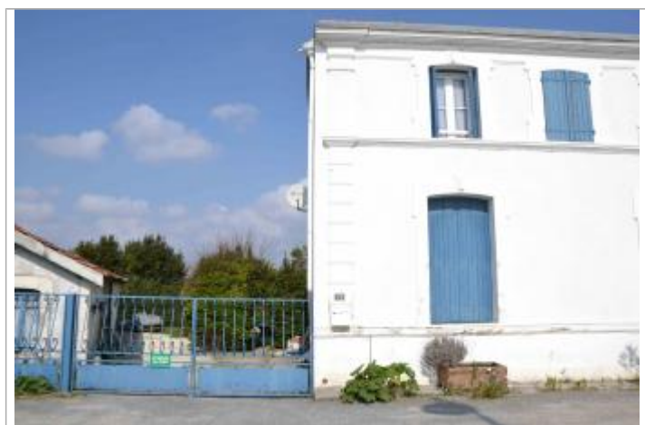
Repère Xynthia place Chatressac
