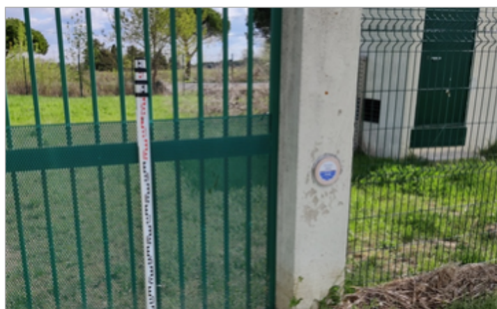
pilier station pompage
