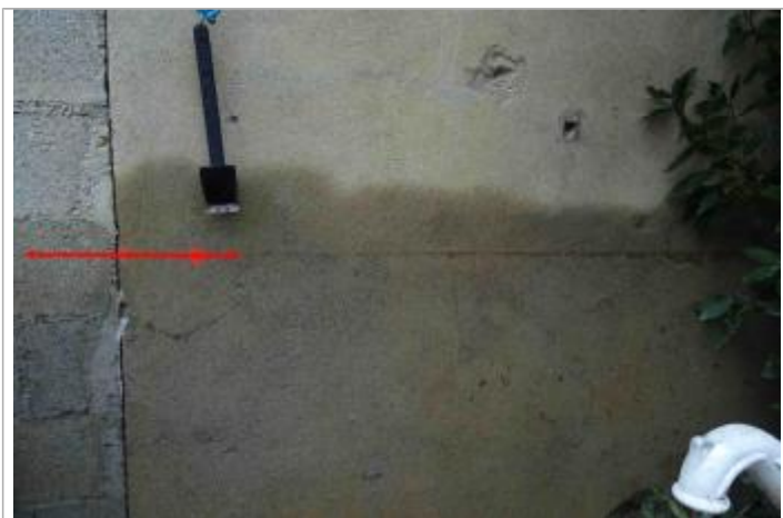
Photo repère © GEOSPHAIR
