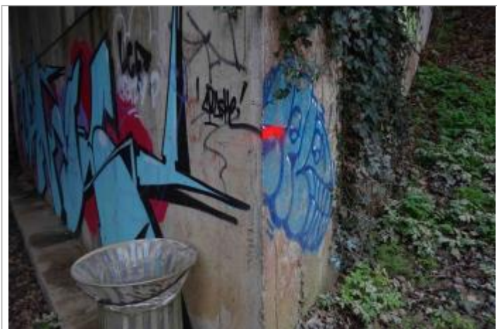
Photo repère © GEOSPHAIR
