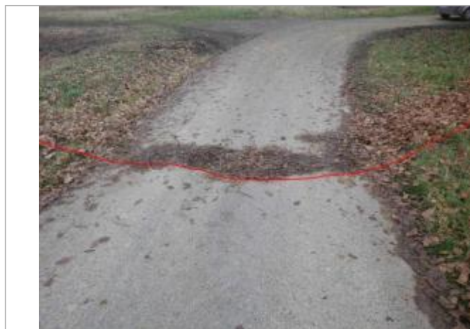
Photo repère © GEOSPHAIR
