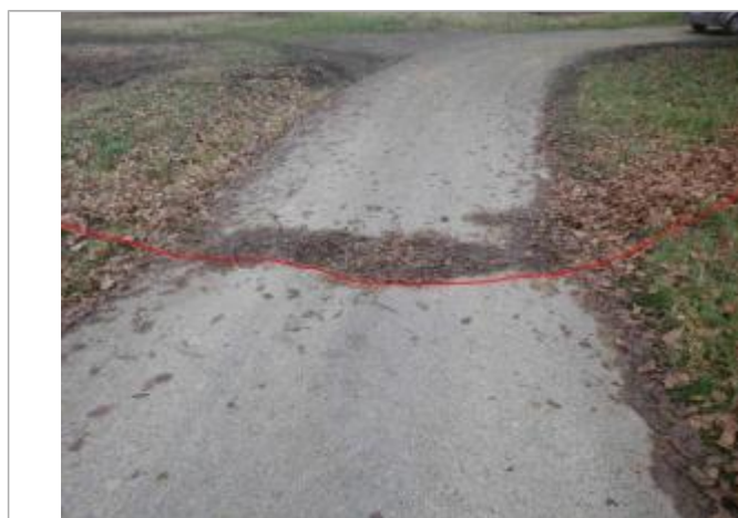
Photo repère © GEOSPHAIR
