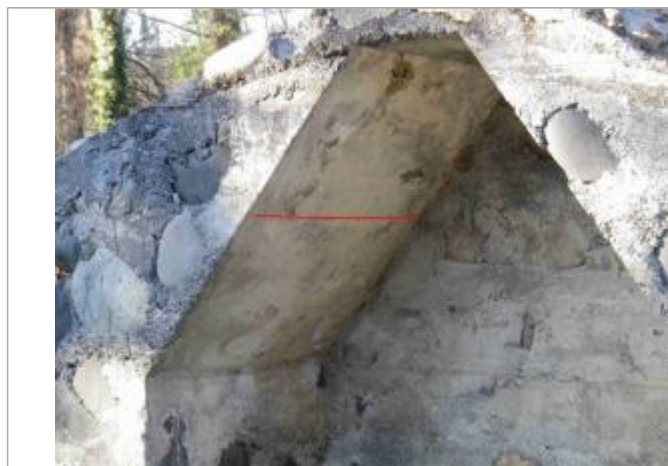
Photo repère © GEOSPHAIR
