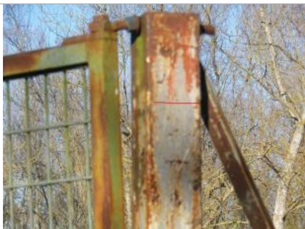
Photo repère © GEOSPHAIR
