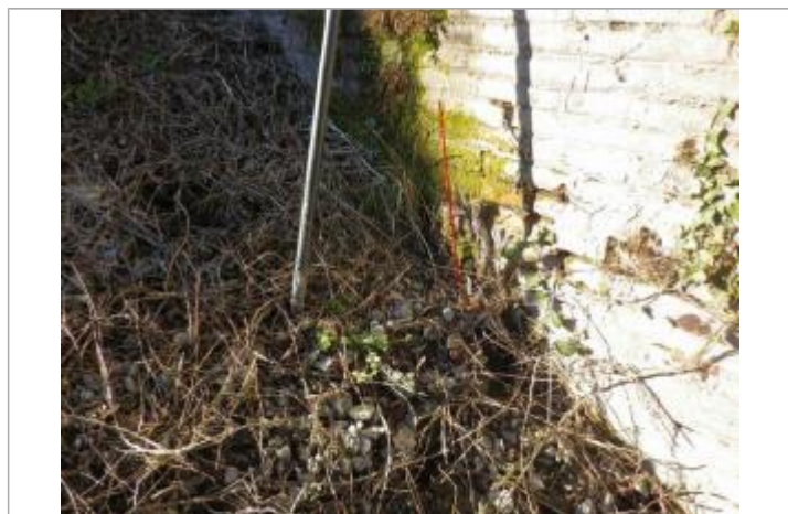
Photo repère © GEOSPHAIR
