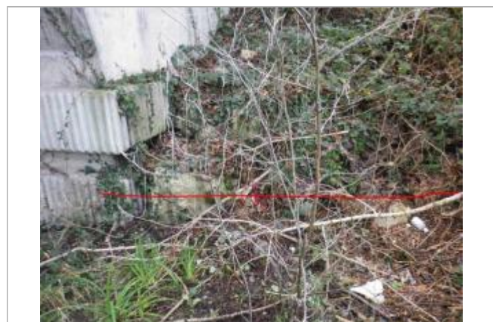
Photo repère © GEOSPHAIR
