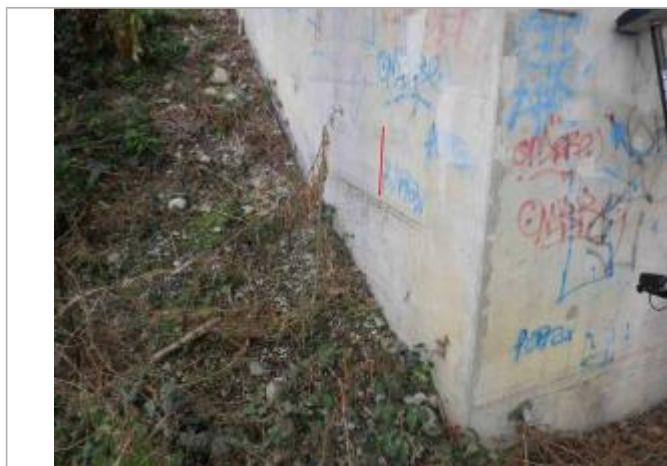
Photo repère © GEOSPHAIR
