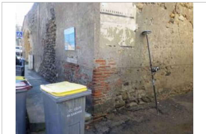
Photo repère © GEOSPHAIR
