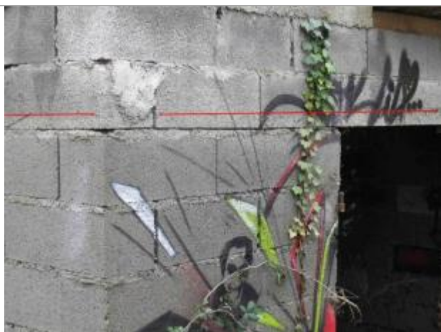
Photo repère © GEOSPHAIR
