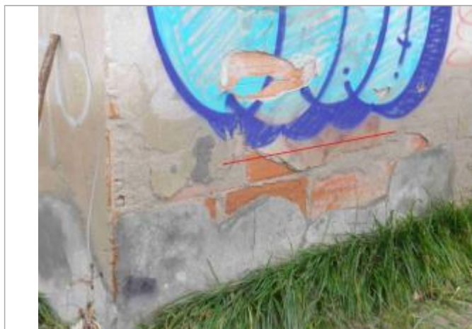
Photo repère © GEOSPHAIR
