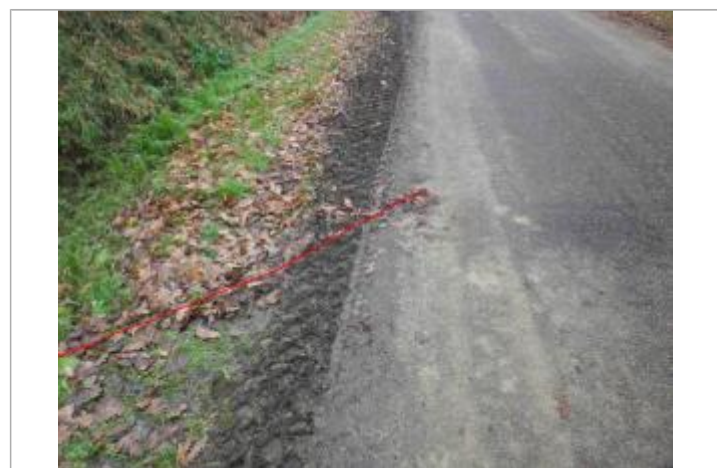
Photo repère © GEOSPHAIR
