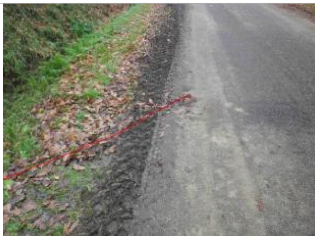
Photo repère © GEOSPHAIR
